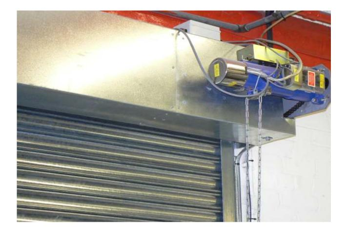
BID Group's Fire Roller Shutters are designed to be robust, providing protection and security whilst providing up to a four-hour delay on the spread of fire in the unlikely event of such a situation. A control desent motor with auto re-set solenoid is fitted as standard.
